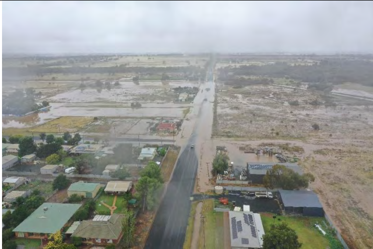
Plate C3.31 – (Photo taken at 13:14 hrs) – Looking south along Wargin Street at its intersection with Blyth Street.
