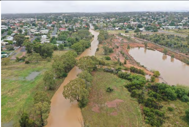
Plate C3.21 – (Photo taken at 12:54 hrs) – Looking west along The Green Corridor from its intersection with Boundary Road.
