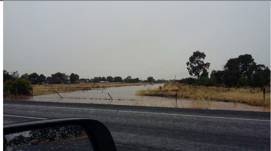
Plate C1.16 – (Photo taken at 10:34 hrs) – Looking east along the Main Drain from Compton Road.
