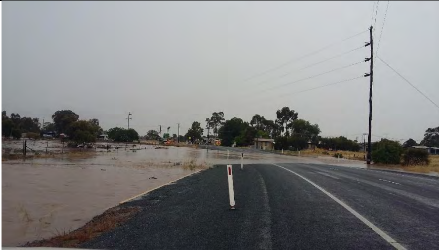
Plate C1.17 – (Photo taken at 11:00 hrs) – Floodwater overtopping Compton Road at low point that is located about 60 m south of its intersection with Cassin Street.
