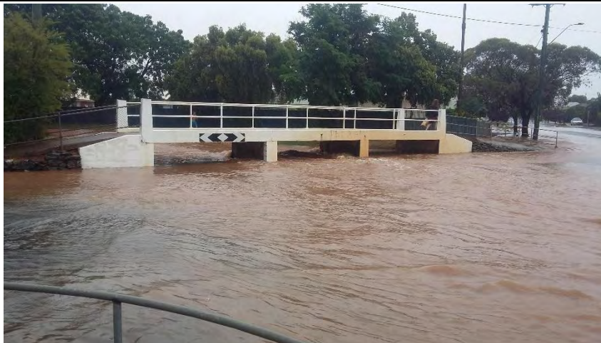
Plate C1.7 – (Photo taken at 10:03 hrs) – Looking west at the footbridge between Barnado Park and Church Street. Depth indicators on bridge indicate floodwater is 200 mm deep.
