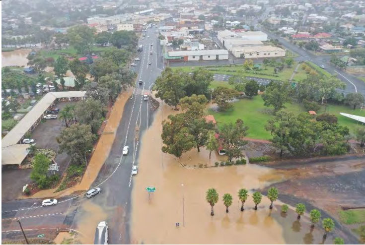
Plate C3.5 – (Photo taken at 11:50 hrs) – Looking east along the Mid-Western Highway from its intersection with Ungarie Road.
