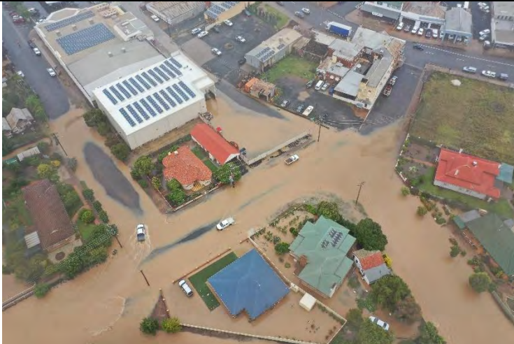
Plate C3.7 – (Photo taken at 11:51 hrs) – Looking south at the intersection of Grenfell Street and Creswell Street.
