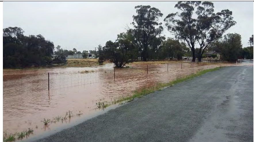
Plate C1.12 – (Photo taken at 10:38 hrs) – Floodwater ponding on upstream (western) side of Sewage Treatment Plant access road.
