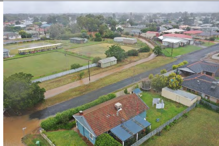
Plate C3.18 – (Photo taken at 12:42 hrs) – Looking north along the channel that runs in a southerly direction on the eastern side of the West Wyalong Bowling Club.
