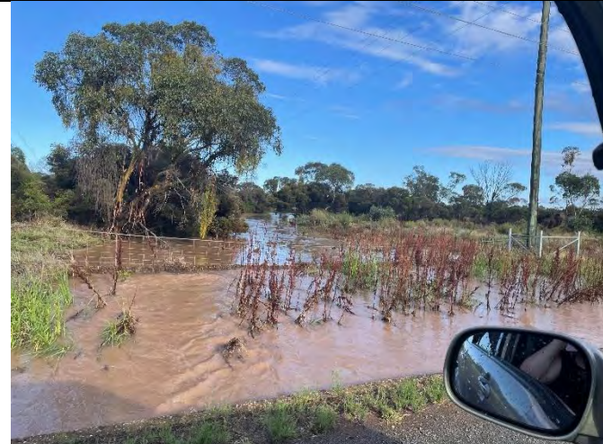
Plate C2.6 - (Time of photo unknown) – Looking west along the Main Drain from Wargin Road.
